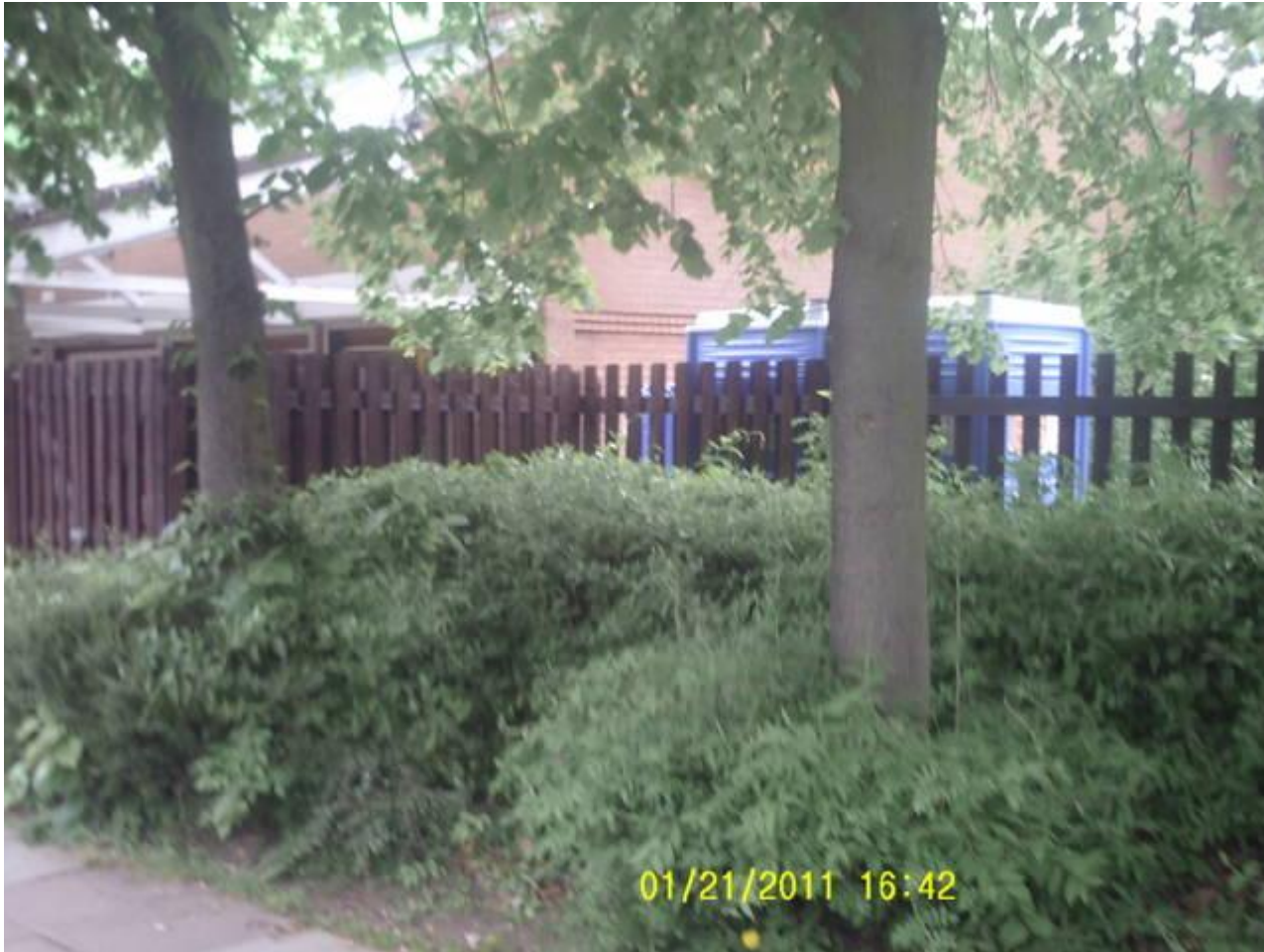
The fencing finished
