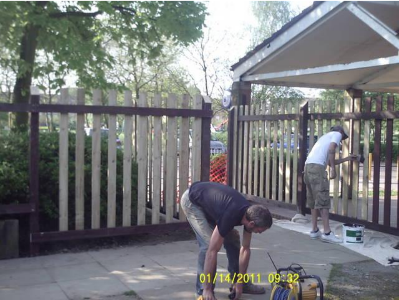
The builders working hard
