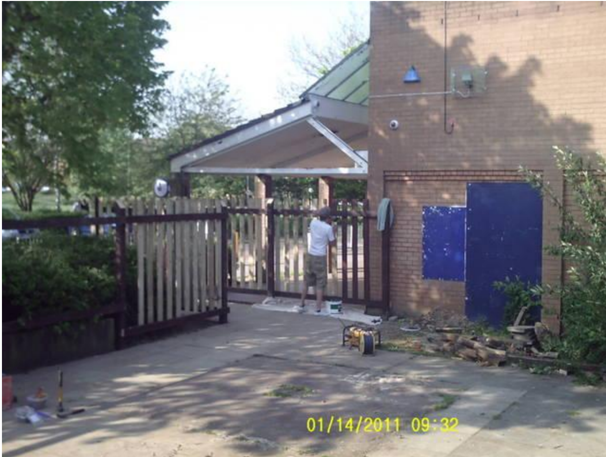
The fencing going up
