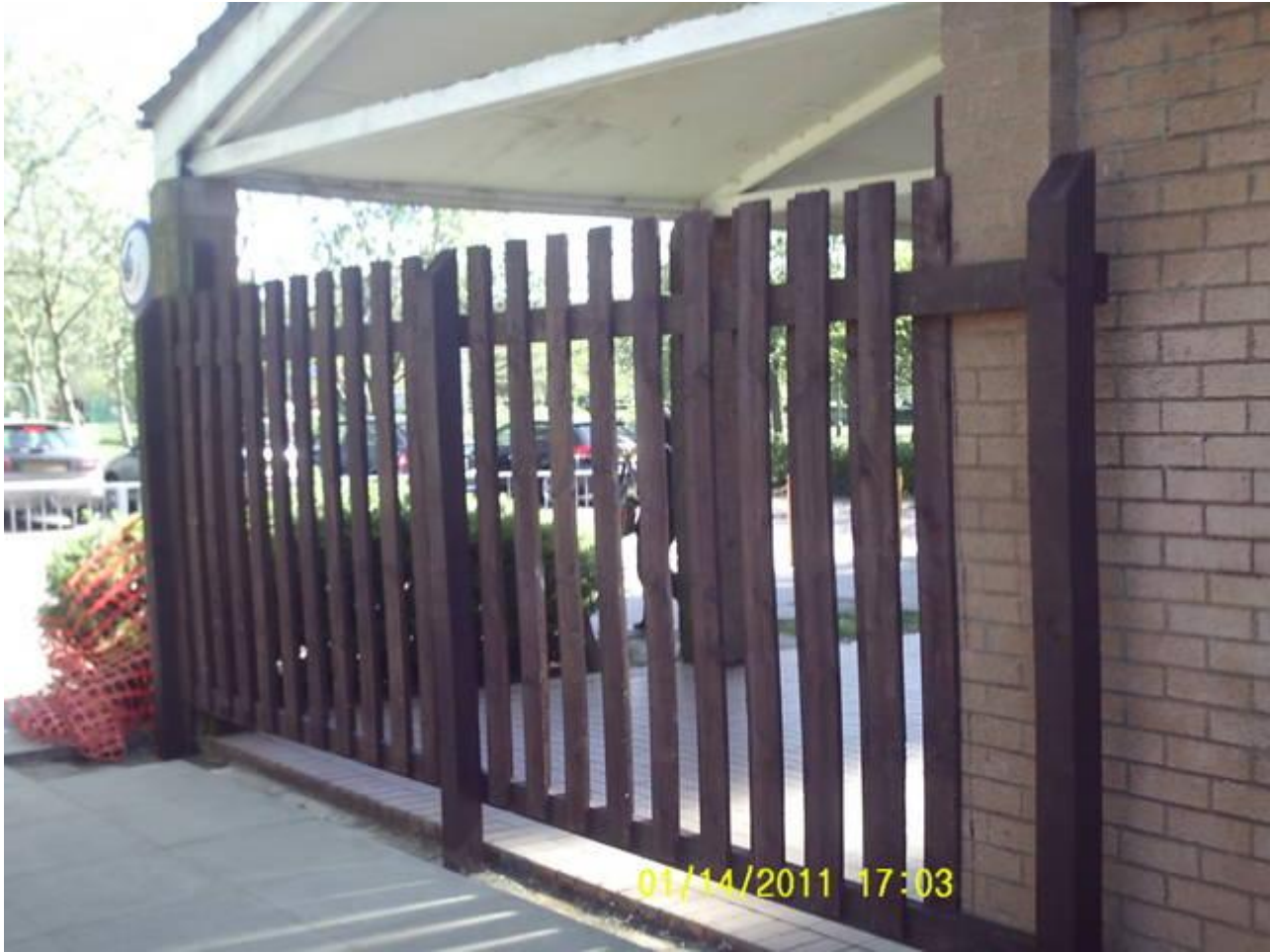
One part complete (Next to the Co-Operative Store)
