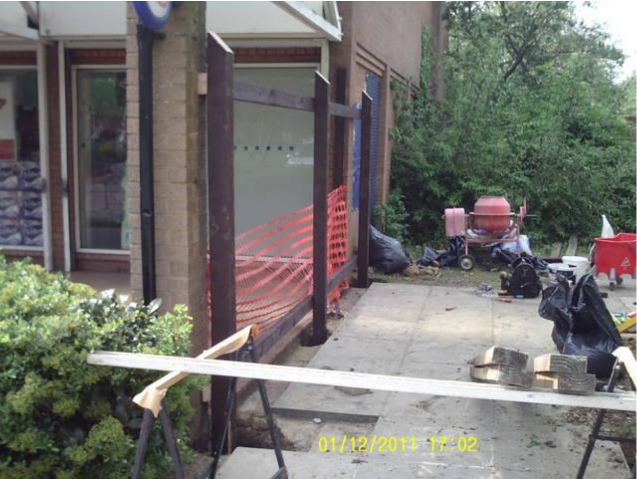
Erecting the fence posts
